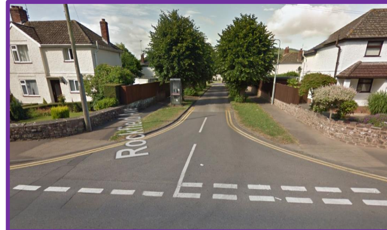
View westwards along Rolls Avenue (from Rockfield Road). The image shows adopted public footway to both sides of the highway, along with traffic calming measures and drop kerbs with tactile paving.
